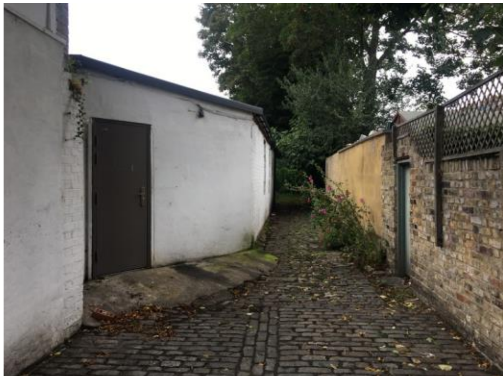
Image 5: Photo of existing application site building
