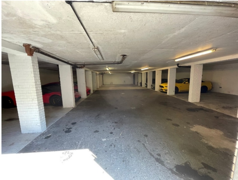
Image 5: Internal Garage Space
