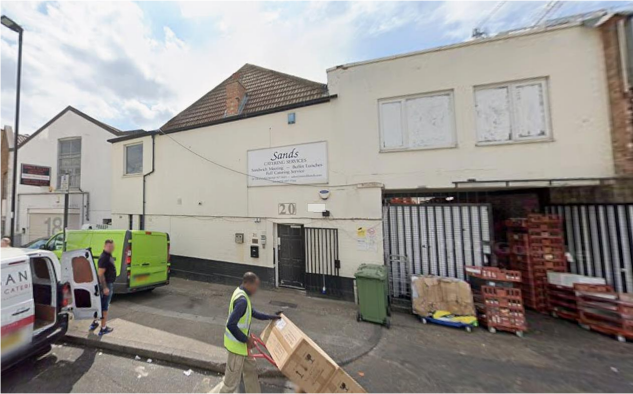
Image 3.4: View of building's front / street elevation (No. 20 Tileyard Road)
