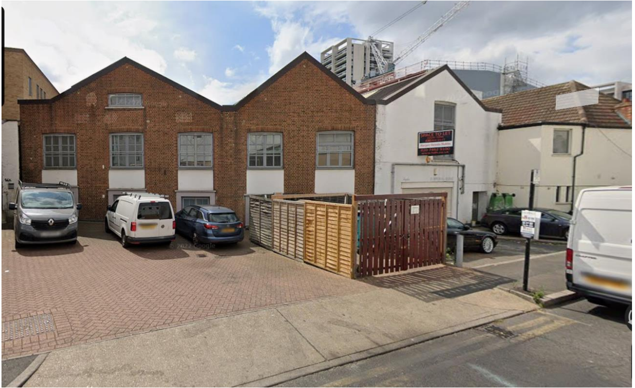
Image 3.3: View of building's front / street elevation (No.18 Tileyard Road)
