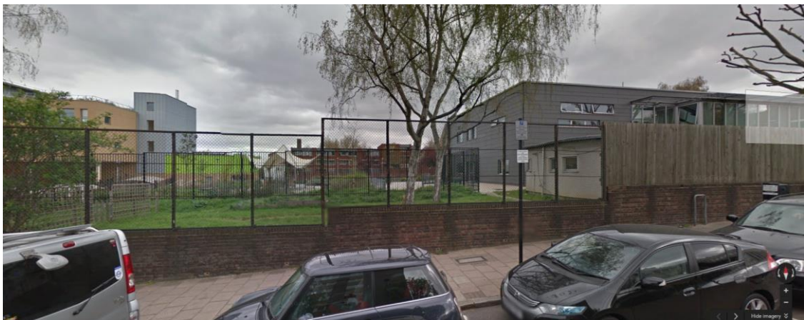
Image 2 Looking at the looking of the location of classroom pod from Donegal Street
