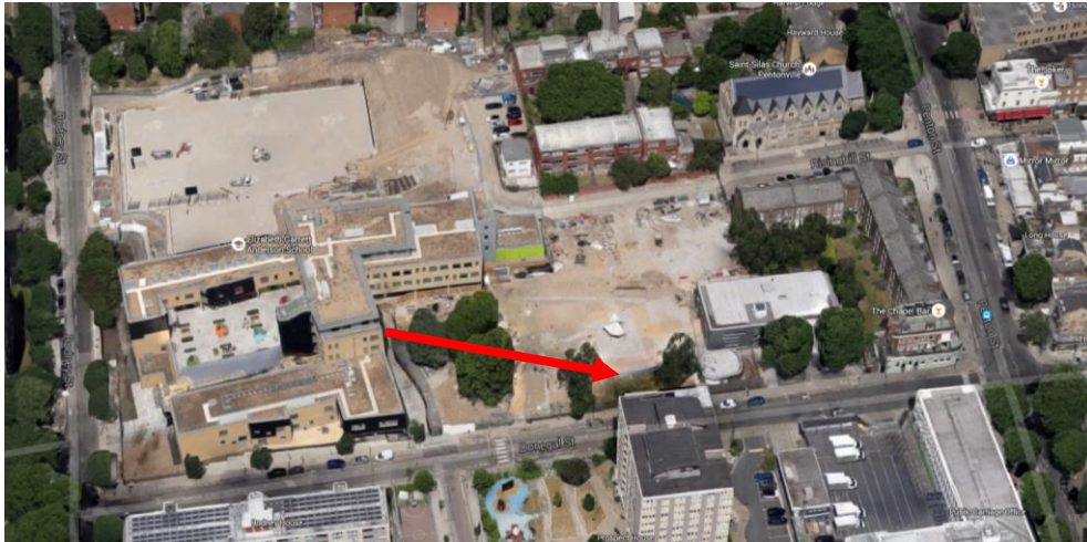
Image 1: Aerial view of the site arrow pointing at location of classroom pod.
