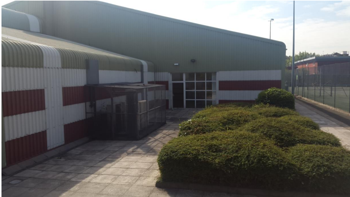
Image 2: Site of proposed plant enclosure
