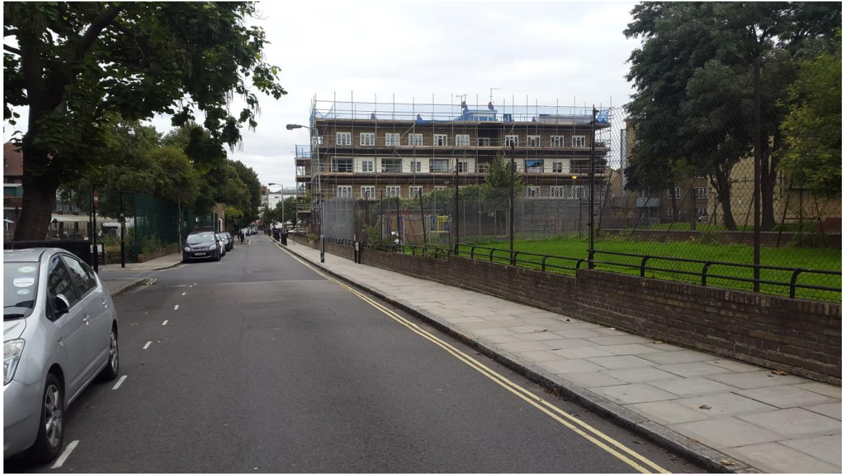
Image 2: View of existing site looking down George's Road to the east
