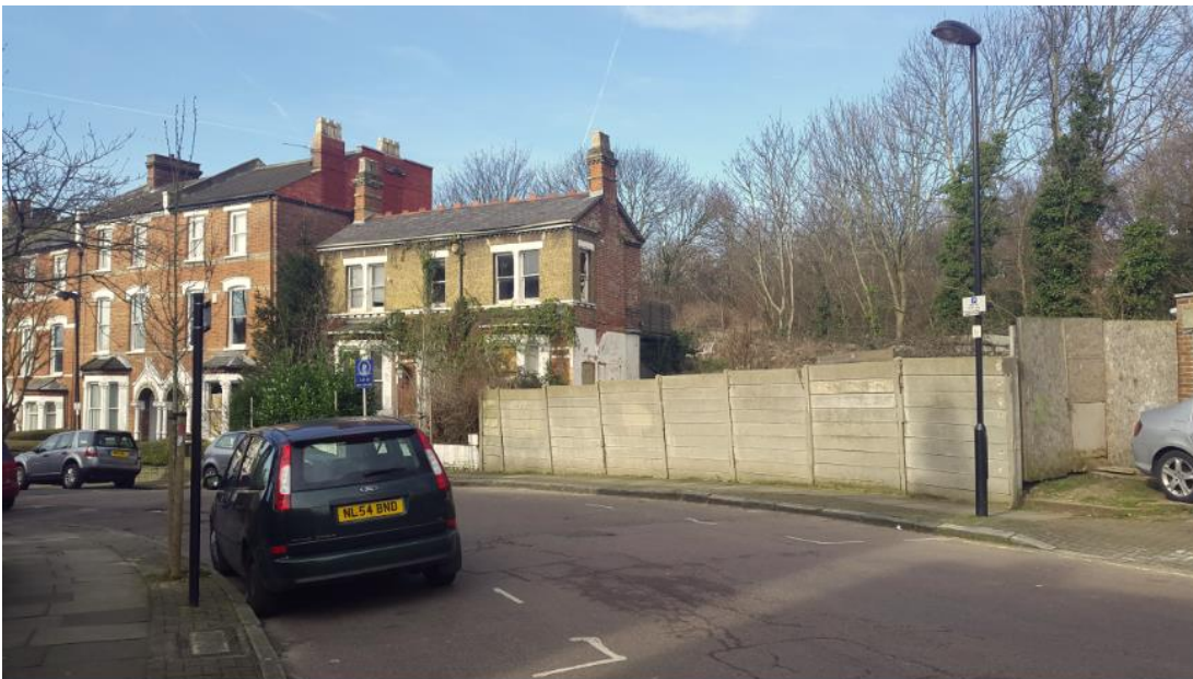
Image 1: The existing building from Blythwood Road
