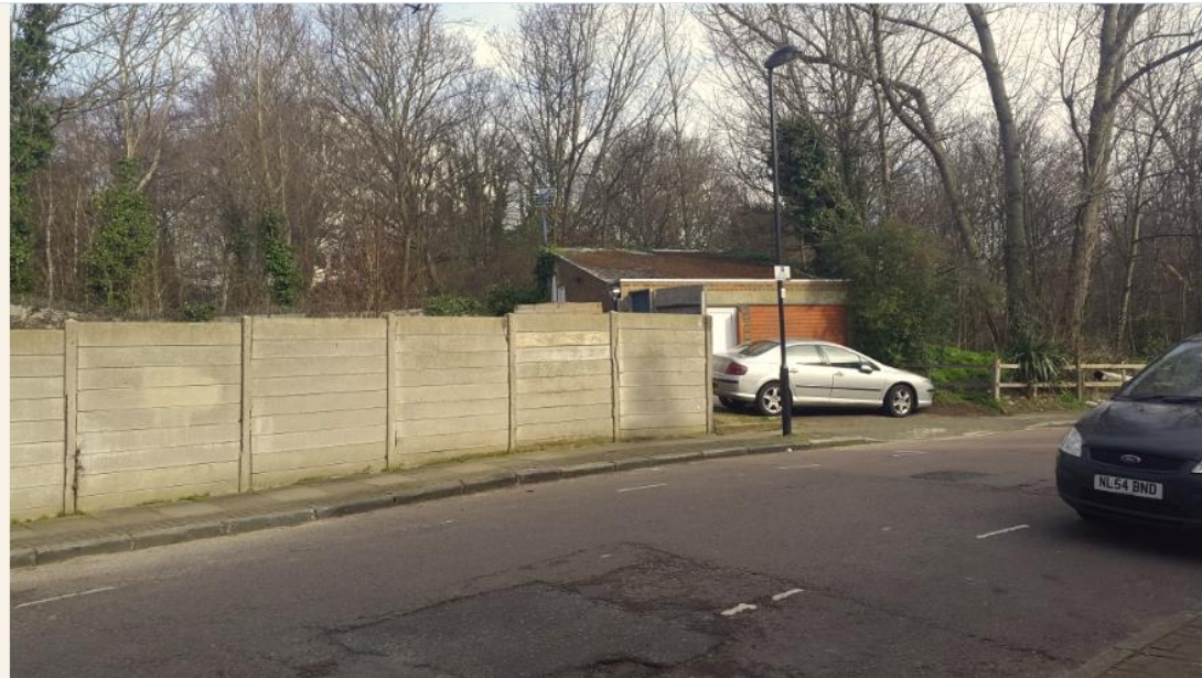
Image 2: Application site viewed from Blythwood Road
