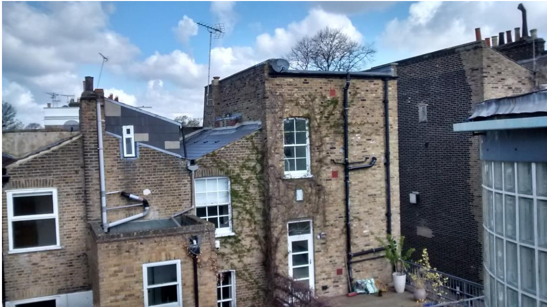
Image 4: View from roof terrace toward properties at Arlington Avenue
