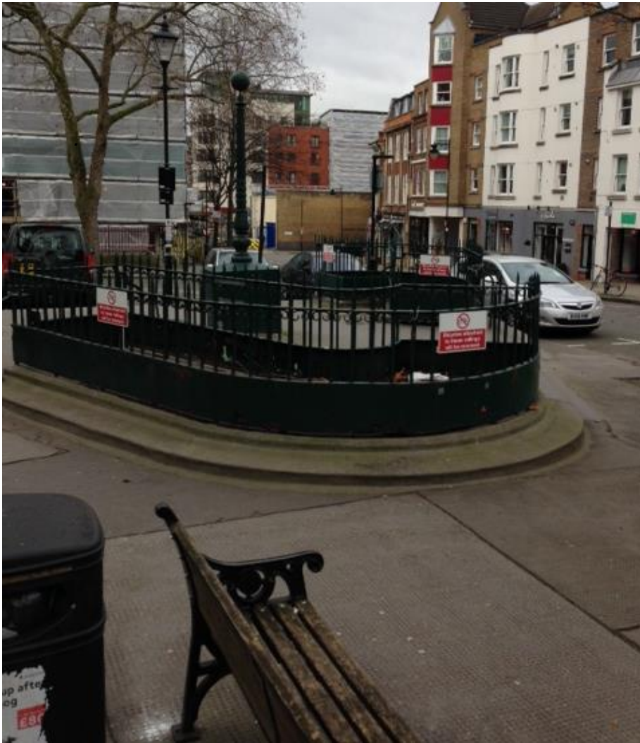
Image 3: view looking north east to the Former Public Convenience
