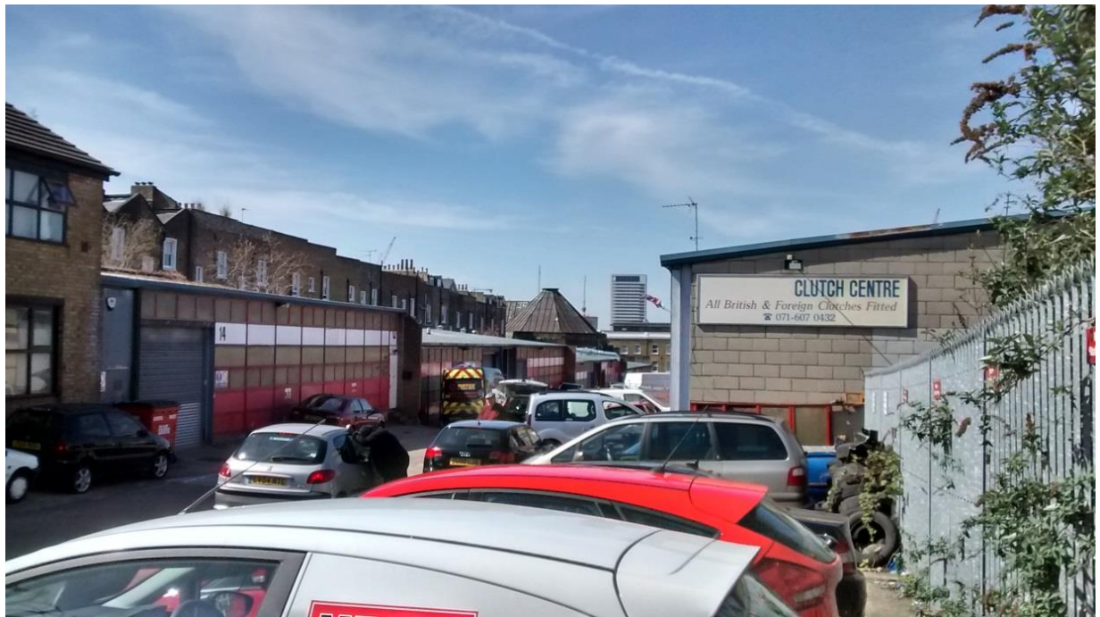
IMAGE 1: Photograph of the site from the entrance to the roman way industrial estate to the east
