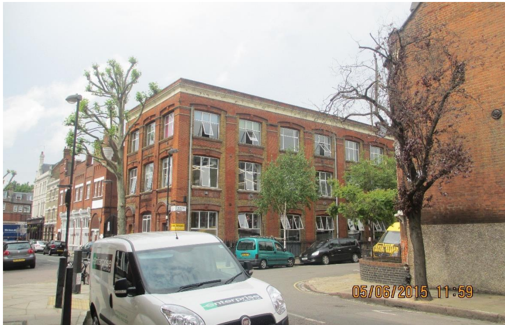
Image 2: Photograph of the application building taken from Ronalds Road looking west.
