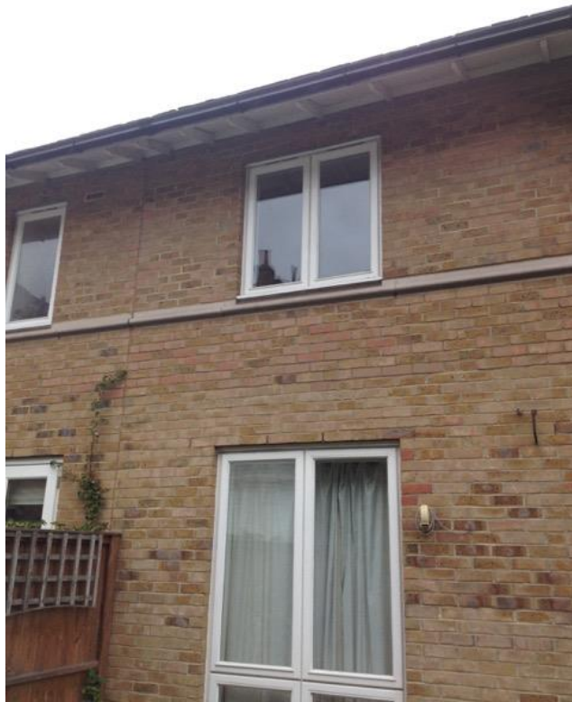
Image 3: View of right side of rear elevation
