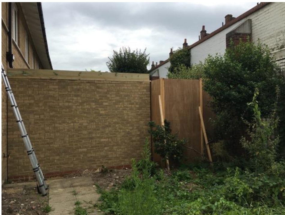
Image 6: View of works to no. 16
