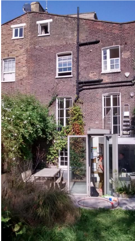
Image 2: Site Photograph showing rear elevation of building
