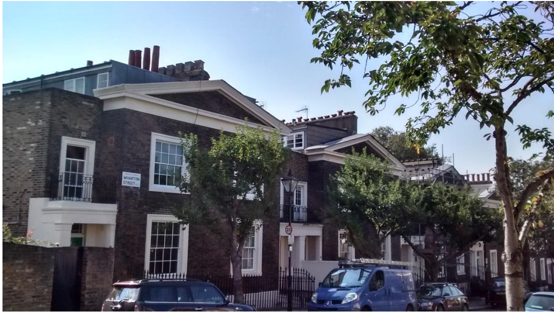
Image 4: Photograph showing front elevation including dormer
