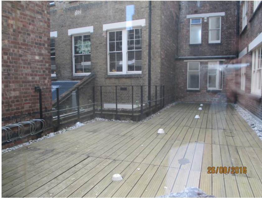
Image 5: Existing terrace above ground floor flat roof
